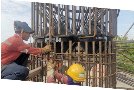
Batang Lupar Bridge, Sarawak BP2500, 16000tn
