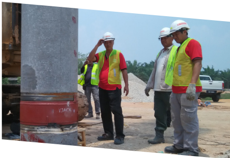
Lekir Village (WCE) SC600, 420tn
