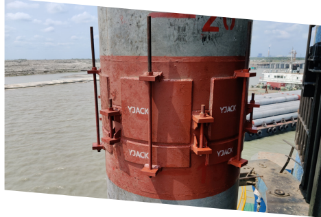
Batang Lupar Bridge, Sarawak SC1000, 840tn
