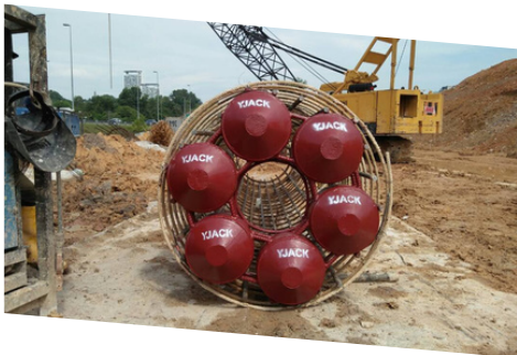
MEX II Expressway, BP1000, 1600tn
