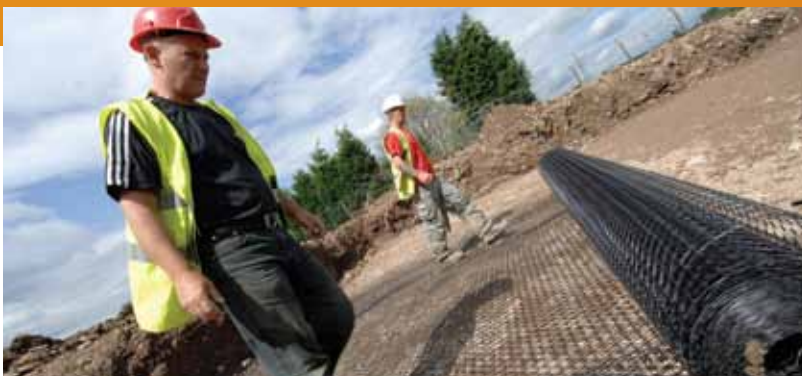
TriAx installation, Stoke
