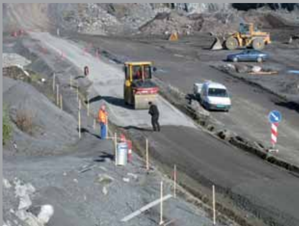
2004 – One of the longest monitored and severely trafficked trials took place in the Feiring Bruck Quarry, Norway
