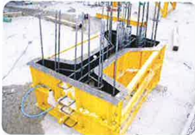
Fabricating the splice block
