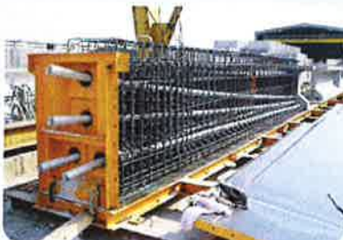
Fabricating rebar and sheath
