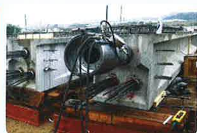
Assembly and prestressing
