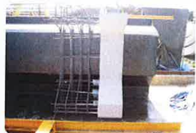
Place a splice block in the form
