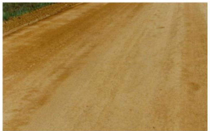
Job done. Very tight and stable surface that will not unravel like ordinary gravel roads do.
