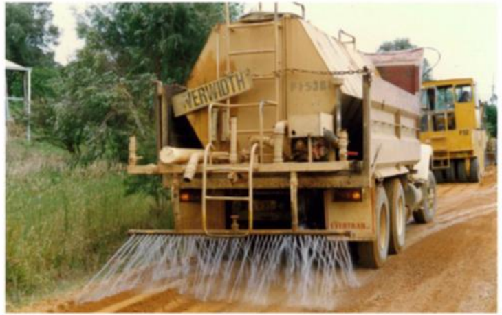
Claycrete™ product mixed with water and disbursed onto soil prior to grader mixing.
