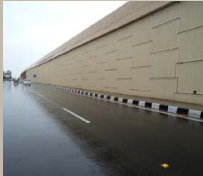
Flyover at ISCON, Ahamdabad, Gujarat, India
