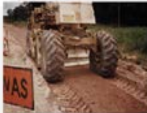
Mixing by Stabilizer
