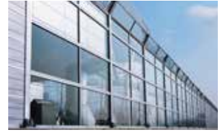
ROAD SAFETY NOISE BARRIER
