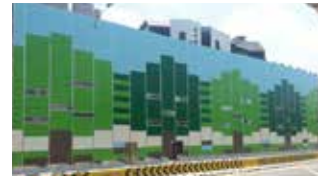
TEMPORARY CONSTRUCTION TEMPORARAY NOISE BARRIER
