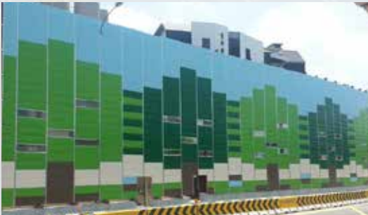
Temporary Noise Barrier
