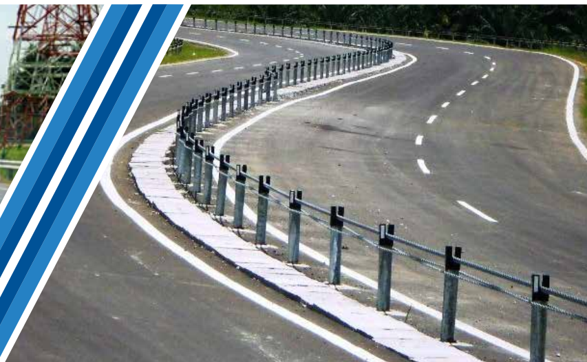
Median and verge installation at curves in Gua Musang, Kelantan
