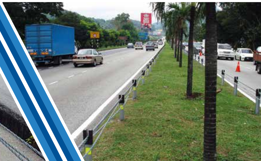
Median installation at Middle Ring Road II, KL
