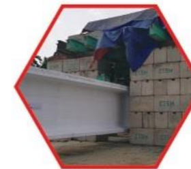
Installation of kentledge
