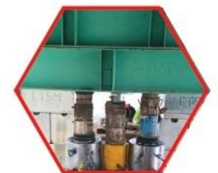
Hydraulic jack and load cell
